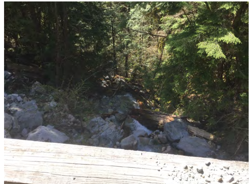
Looking downstream from deck
