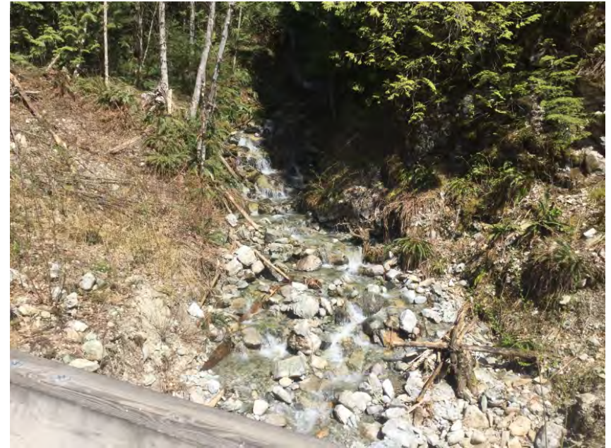
Looking upstream from deck
