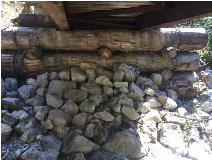
Left Bank Abutment when facing downstream
