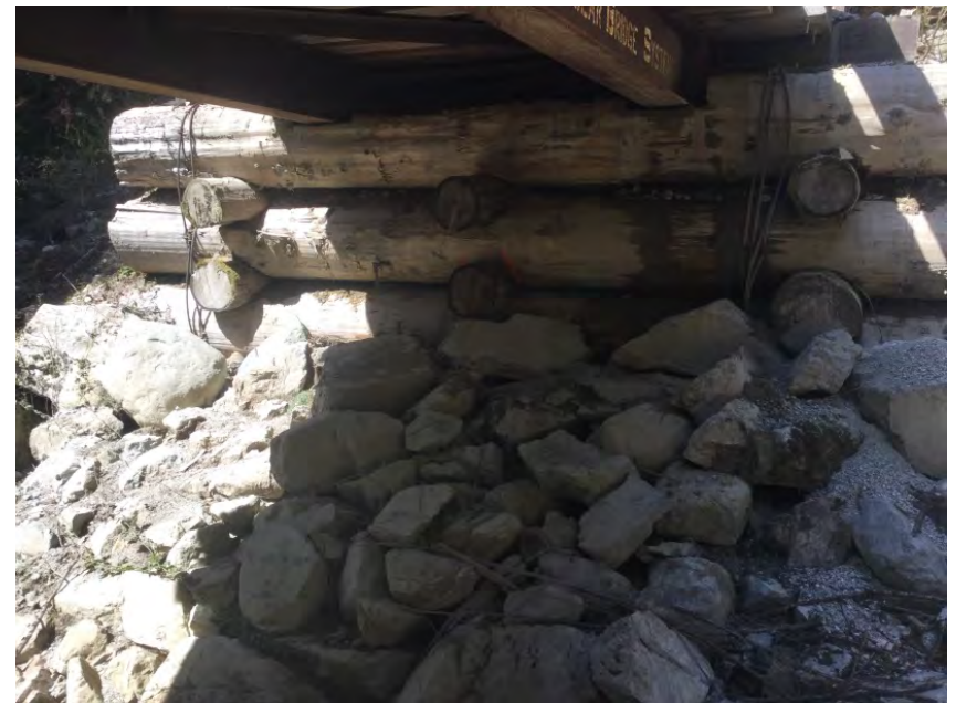
Right Bank Abutment when facing downstream
